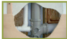
SERVICES DUCT BETWEEN ALL CASSETTES FOR PLUMBING, WASTE, ELECTRICS, HEATING AND VENTILATION
